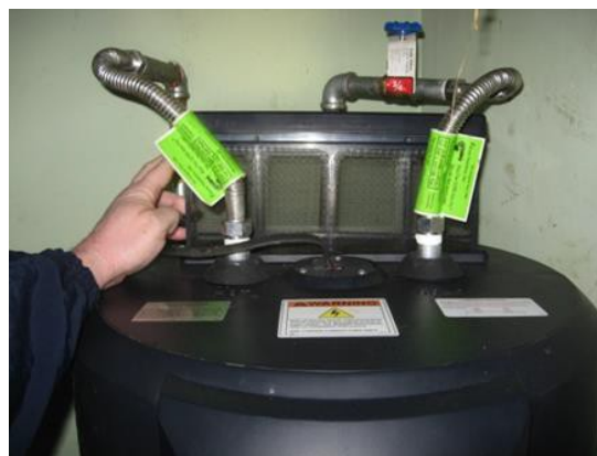
Figure 4.14. GE heat pump water heater filter.
