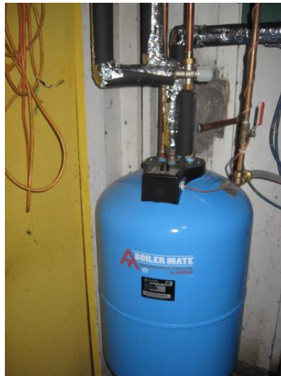
Figure 4.17. Indirect water heater with removable heat exchanger and external mixing valve.
