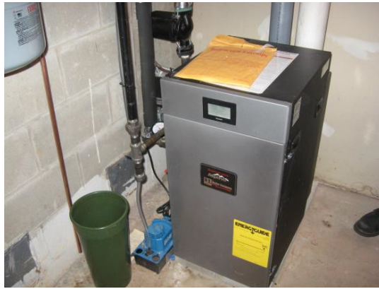
Figure 4.16. Gas condensing boiler— 96% annual fuel utilization efficiency.
