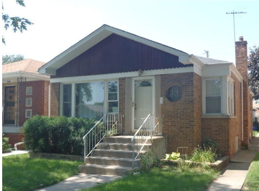
Figure 4.22. Example of a masonry home in Chicago, Illinois.
