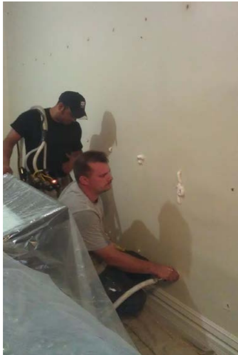
Figure 4.23. Injecting masonry foam into wall cavities.
