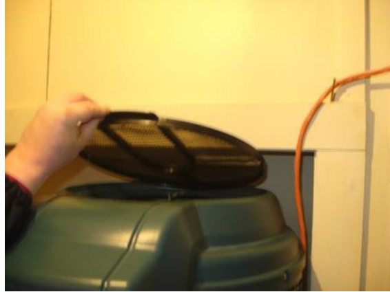
Figure 4.15. Rheem heat pump water heater filter.
