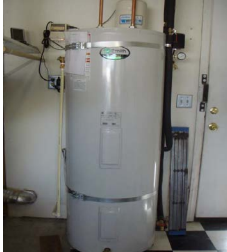
Figure 4.6. Solar water heater water storage tank.
