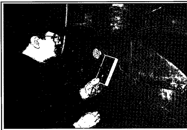
This manometer is a precision instrument that can be used as both a draft gauge (shown with a large boiler) and as a tool to explore air leakiness between zones and stack-effect infiltration.
