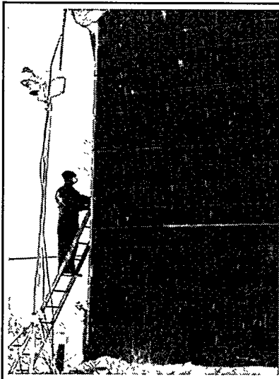
Installing insulation as the snow flies.
