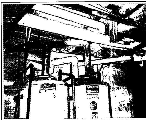
The weatherization crew which insulated the tank and pipes entering and exiting from this hot water heater did an excellent job.
