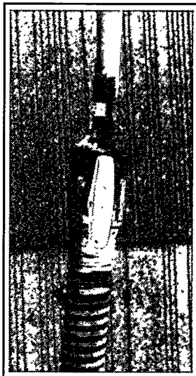
The small tube at the top is snaked into wall cavities, then slowly withdrawn as insulation fills them up. The result is a very tight fill.
