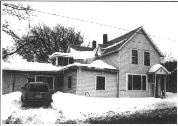
Patterns of snow and ice indicate a leaky, poorly insulated attic.
