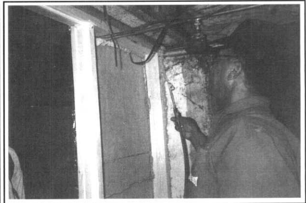
Sealing a new basement partition wall.
