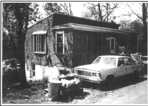
The weatherization job on this house will include foundation wall repair.
