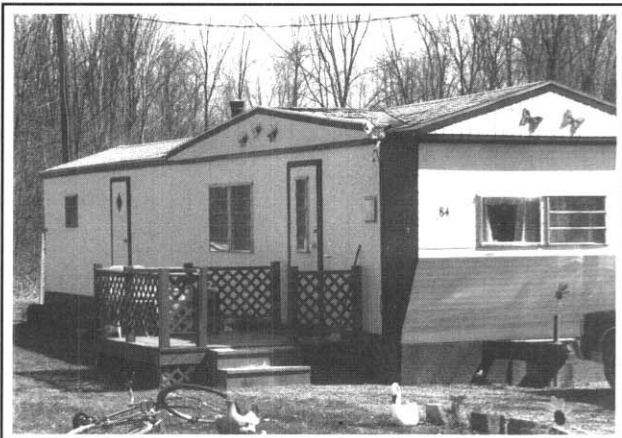
Skirting under a mobile home is not as important for the heating bill as belly board insulation, which can be blown in by weatherization crews.
