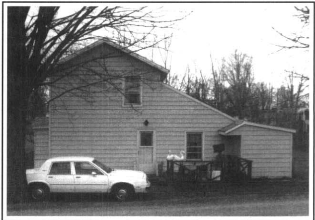
This roofline suggests complex paths for air leakage.
