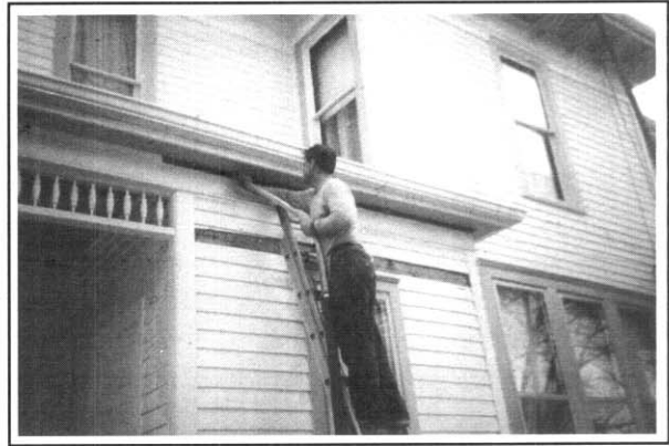
As revealed by a blower door and a pressure gauge in a test that takes only several minutes, the area under this porch is directly connected to the envelope through floor joists between the first and second floor. High-density insulation is being used to air-seal this largest hole in the dwelling.
