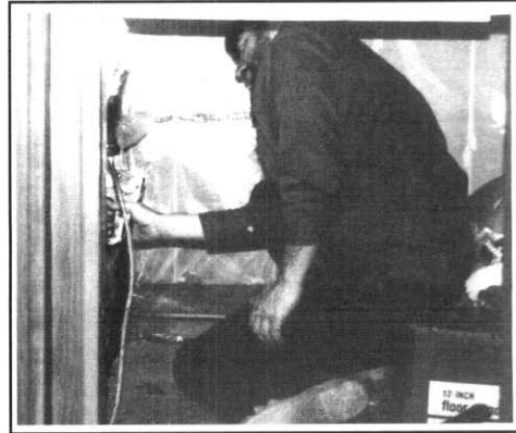
Air sealing a plumbing chase on the first floor that corresponds with both attic and basement. Sealing holes in inconspicuous and hard-to-get-to places are frequently those which result in good, cost-effective weatherization jobs.
