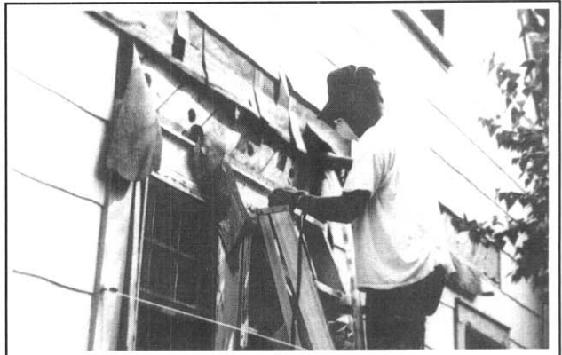
Wall preparation. Shingles are positioned for fast reattachment after insulation blowing.
