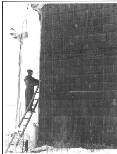
Installing insulation as the snow flies.
