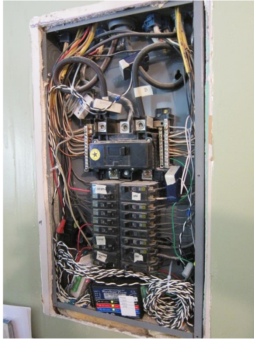
Fig. 2. Panel-level metering equipment located inside the home's main electric panel (Site 6).
