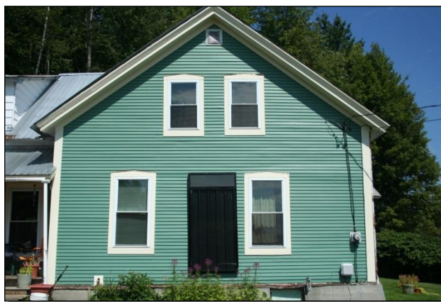
Fig. 9.4. Solar Hot Air Panel (between two first floor windows)
