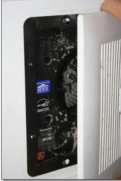
Fig. 8.9. Panasonic Whisper bathroom ventilation fan
