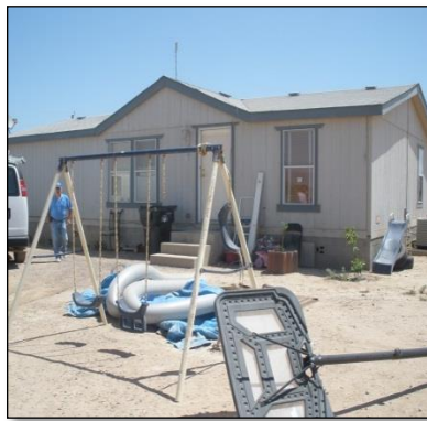
Fig. 7.2. Trailer without shade, in hot/dry climate
