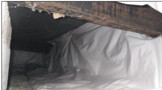
Fig. 3.6 Insulation viewed from underneath the mobile home.
