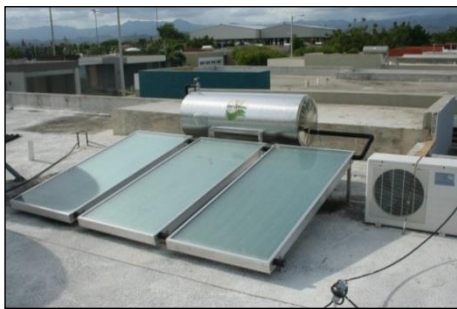
Fig. 2.16. Solar water heaters
