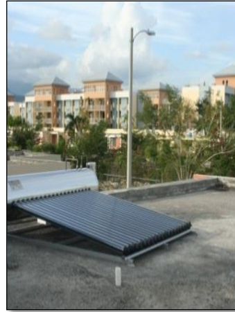
Fig. 2.19. Roof Solar HW Heater
