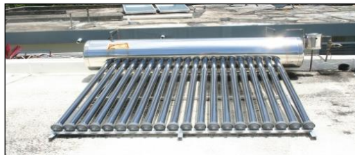
Fig. 2.4. Solar Water Heater
