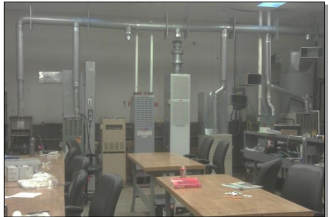
Fig. 10.3. HVAC training center- various heating systems
