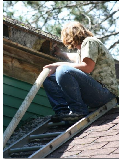
Fig. 9.7. Blowing insulation into access holes cut into ridge
