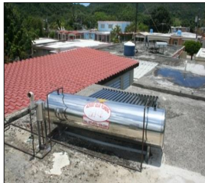
Fig. 2.8. Roof Solar HW
