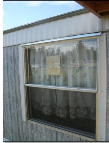
Fig. 5.8. Flashing above a window and around the perimeter of a mobile home
