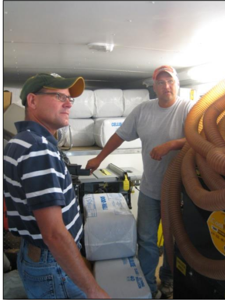
Fig. 15.2. Weatherization Staff and Supplies
