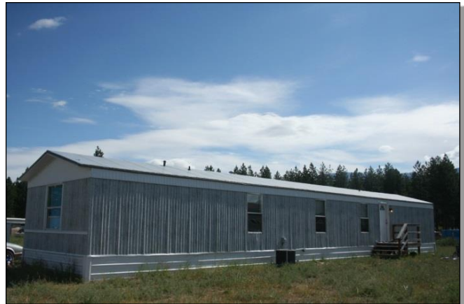
Fig. 5.5. Weatherized mobile home in SKHA’s 80-lot trailer park
