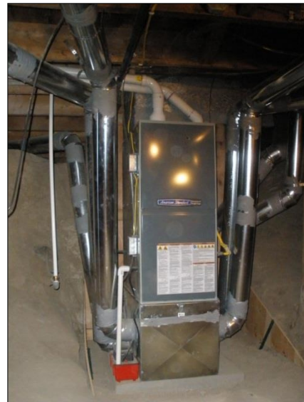
Fig. 3.10. New energy-efficient furnace installed in crawl space with new duct work.
