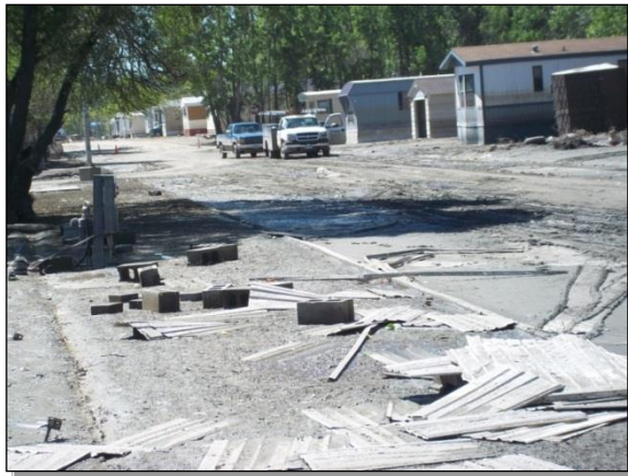
Fig. 15.11. Minot housing stock after the flood
