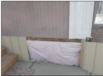
Fig. 3.5 Burrito insulation viewed from side of mobile home.
