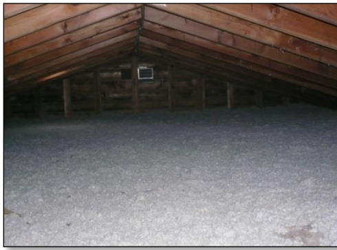
Fig. 12.1. Insulation in the attic protects the living space from cold.
