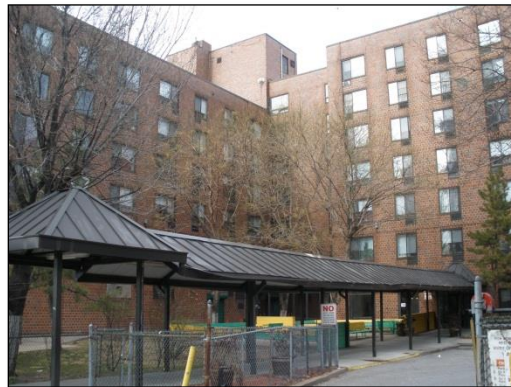
Fig. 13.11. Senior Citizen home weatherized by AEA. (Note: Upper-floor windows are closed, which is indicative of uncomfortable heat distribution. Uneven heat distribution is a common issue with MF buildings).
