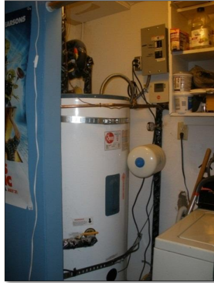
Fig. 6.7. Solar water-heater tank
