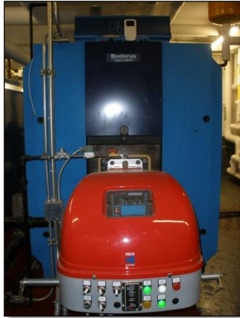
Fig. 13.7. Boiler installed by AEA
