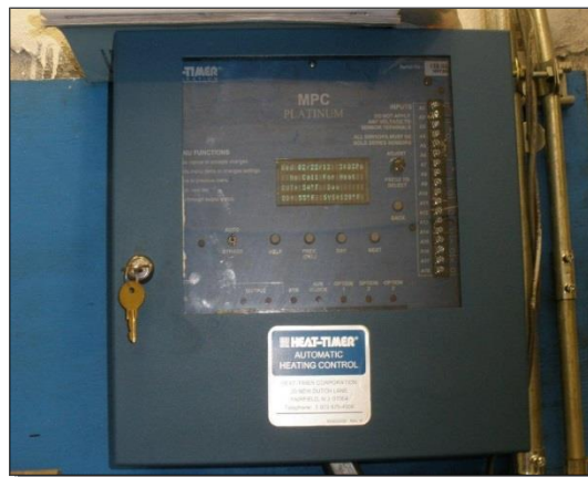
Fig. 14.5. Heating System Controls
