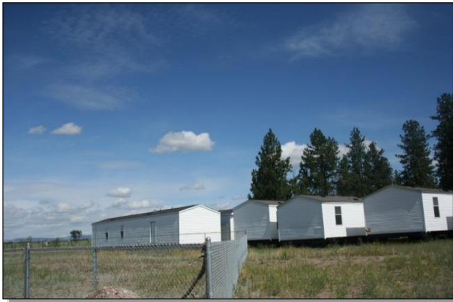
Fig. 5.4. FEMA Trailers Weatherized For Home Ownership
