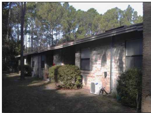
Fig. 11.11. Multifamily apartment house with inverted mini-split unit outside.
