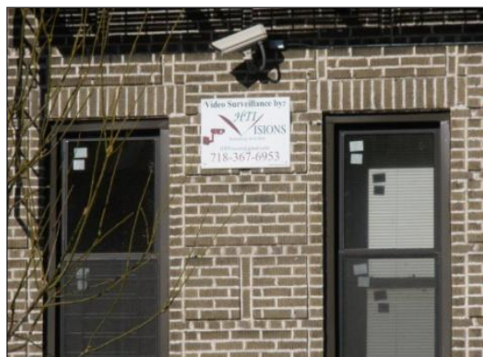
Fig. 14.6. Camera and Surveillance System
