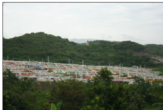
Fig. 2.29. Southwestern housing development with several rooftop solar HW heaters
