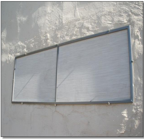
Fig. 6.3. Multifamily unit with solar screens installed (top); close-up of solar screens (bottom)
