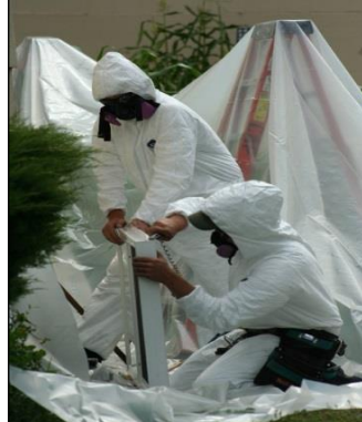
Fig. 4.8. Window replacement crew in full lead protection kit
