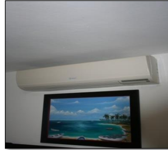
Fig. 2.15. Wall AC unit
