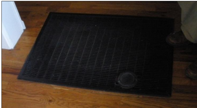
Fig. 3.9. (Pre-weatherization) Grate for sole heat source in residence. Open flames were visible from above.
