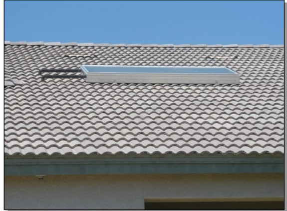
Fig. 7.7. Solar panel for Hot water heater on roof of Women's and children's Shelter
