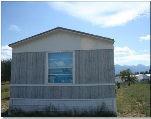
Fig. 5.7. Flashing around the perimeter of a mobile home
