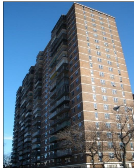
Fig. 16.3. One of seven buildings within Lindsay Park.
