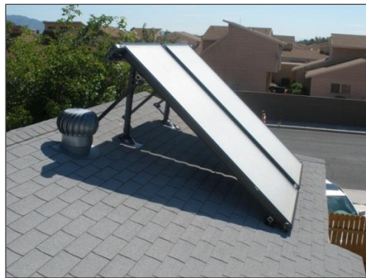
Fig. 6.5. Rooftop solar panels
