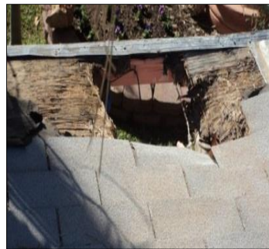
Fig. 7.3. Roof damage
