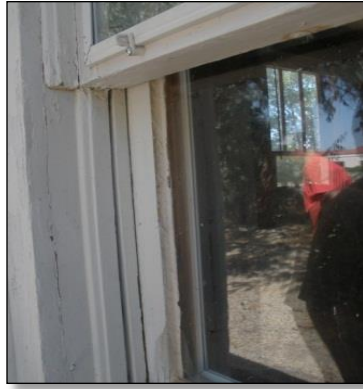
Fig. 3.7. Double-storm window innovation.
