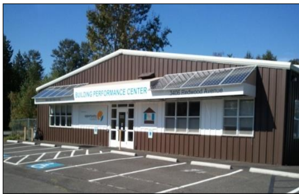
Fig. 8.5. Building Performance Center, the OC's weatherization training facility
