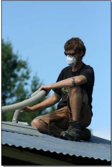
Fig. 9.6. Blown-in Cellulose Insulation
