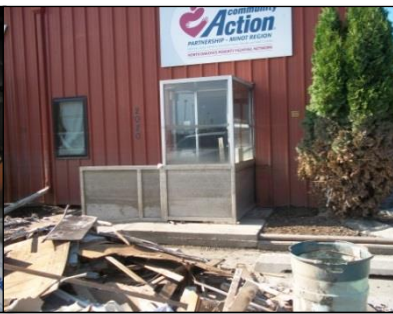
Fig. 15.9. Weatherization Warehouse Flooded
