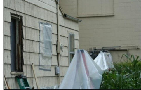
Fig. 4.9. Lead-Safe window replacement with plastic garden barrier
