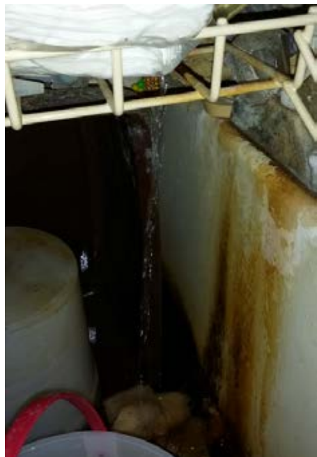
Figure 25. Faucet left running in the winter to prevent frozen water lines.
