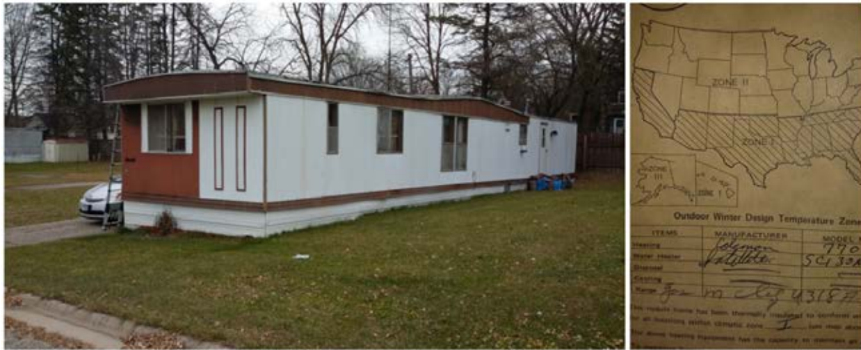
Figure 19. One of two homes in the study carrying a data plate indicating that it is meant to be located in a warmer climate zone.
