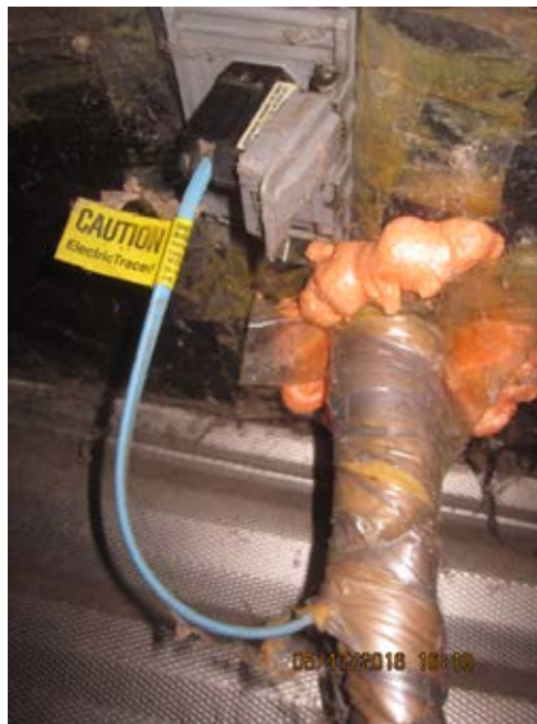
Figure 26. Heat tape installed under pipe insulation.
