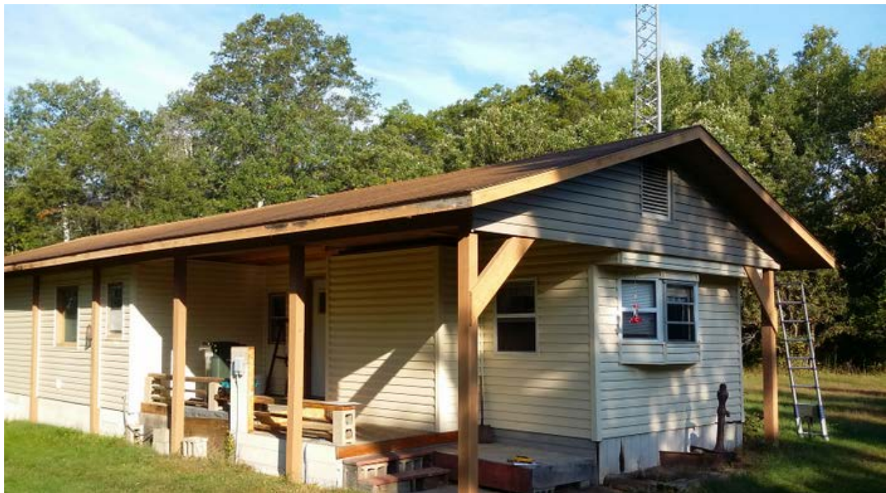
Figure 16. A manufactured home with a separate roof structure built over it.
