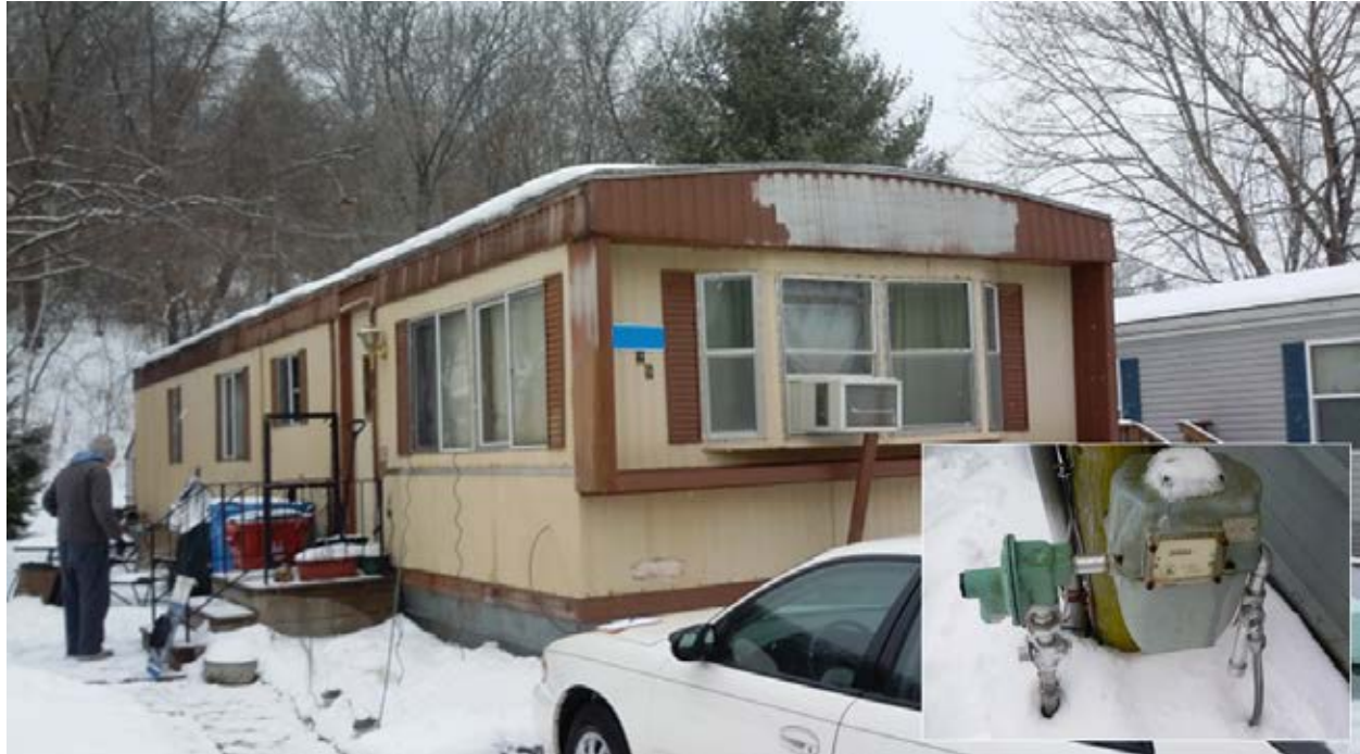
Figure 13. This manufactured home is in a park with a propane sub-metering arrangement (inset photo).
