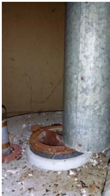
Figure 36. Disconnected water-heater venting.
