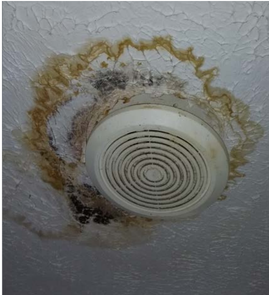
Figure 34. A quiet, continuously-operating bath fan installed by local weatherization agency to meet ventilation requirements.
