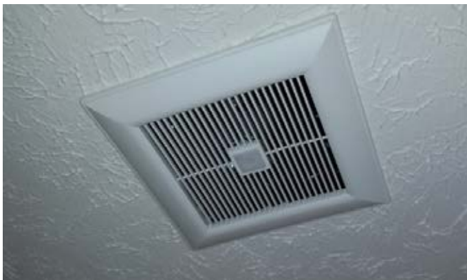
Figure 34. A quiet, continuously-operating bath fan installed by local weatherization agency to meet ventilation requirements.
